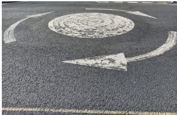
Figure 7: Roundabout – supervisor's control (IIS 1)
