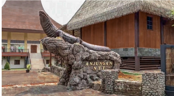
Figure 3: The house shape from NTT Province in TMII
